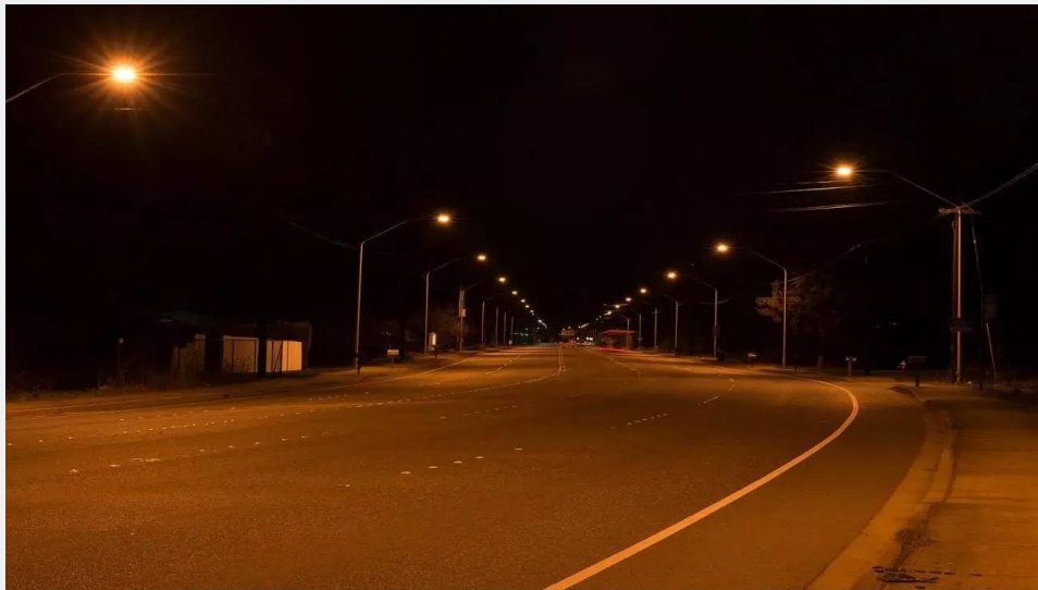
Figure 2: High-Pressure Sodium (HPS) lighting showing a dimmer, yellowish hue.
